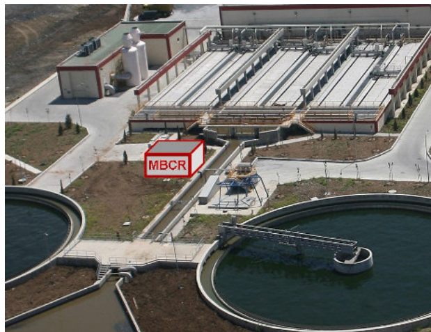
Figure 2: Illustrational mounting of pilot plant on Ataköy WWTP
